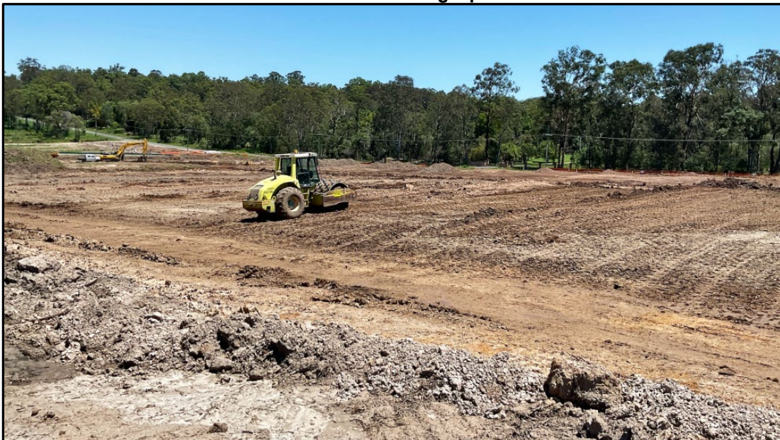
Picture 2: View of Filling Operations
