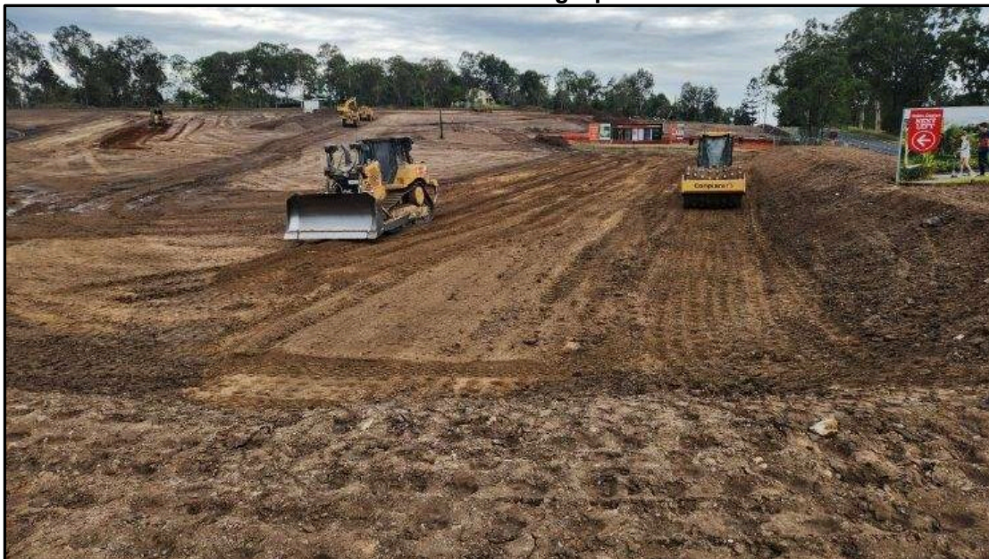
Picture 2: View of Filling Operations
